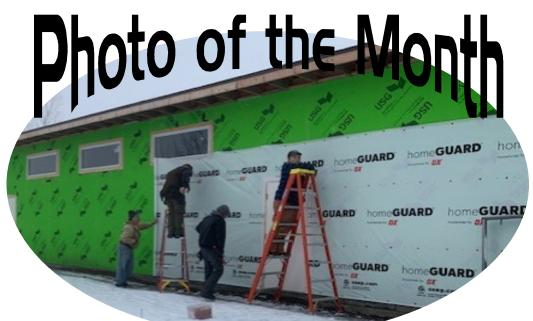
It's a wrap! Josh, Josh, Greg and Steve are working here. Another crew worked during the Ladies' Tea, and two old guys on a lift finished the high parts. All the soffit and fascia are up, the building is wrapped, and we're good until spring, when it's time to put on the siding!
